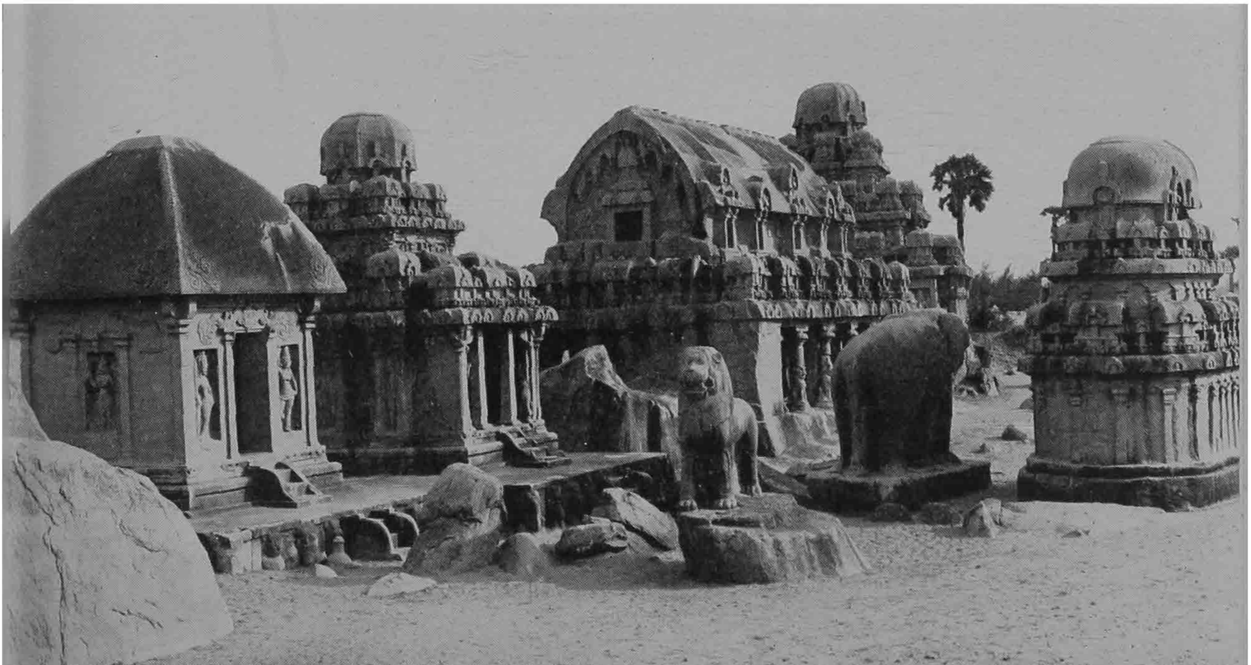
The 'Raths' of Mahābalipura. (Photo: Archaeological survey of India, Southern circle)
