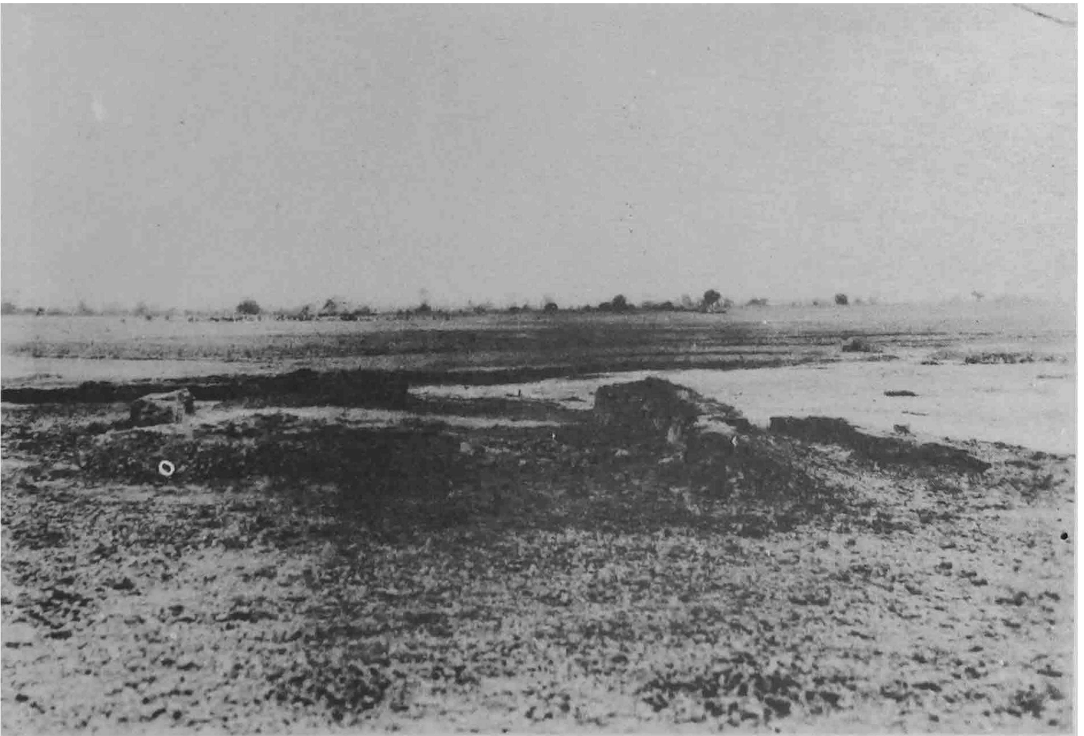
b. Remains of structure at KKG 21.
