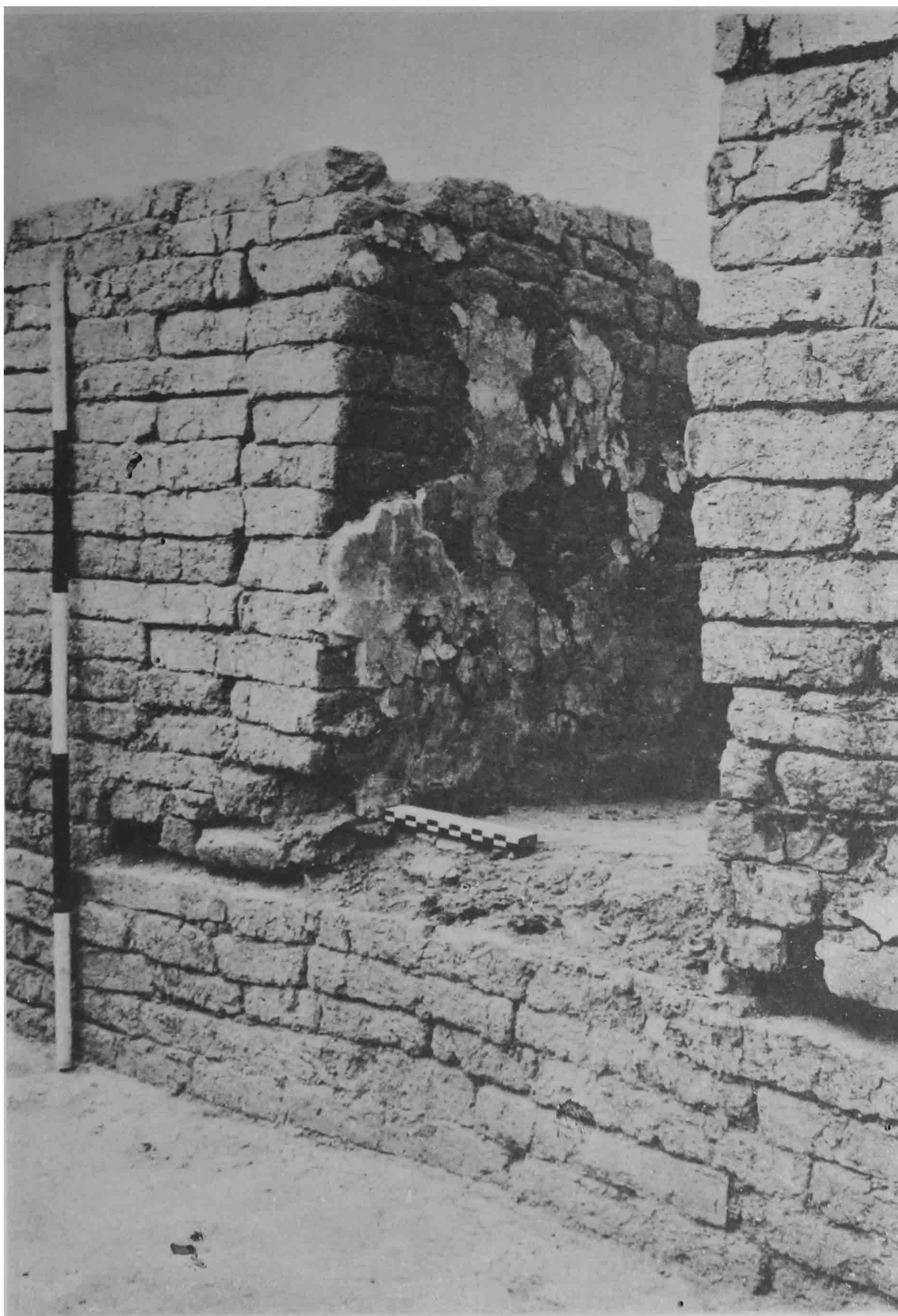
One of the windows in the structure, KKG 2.
