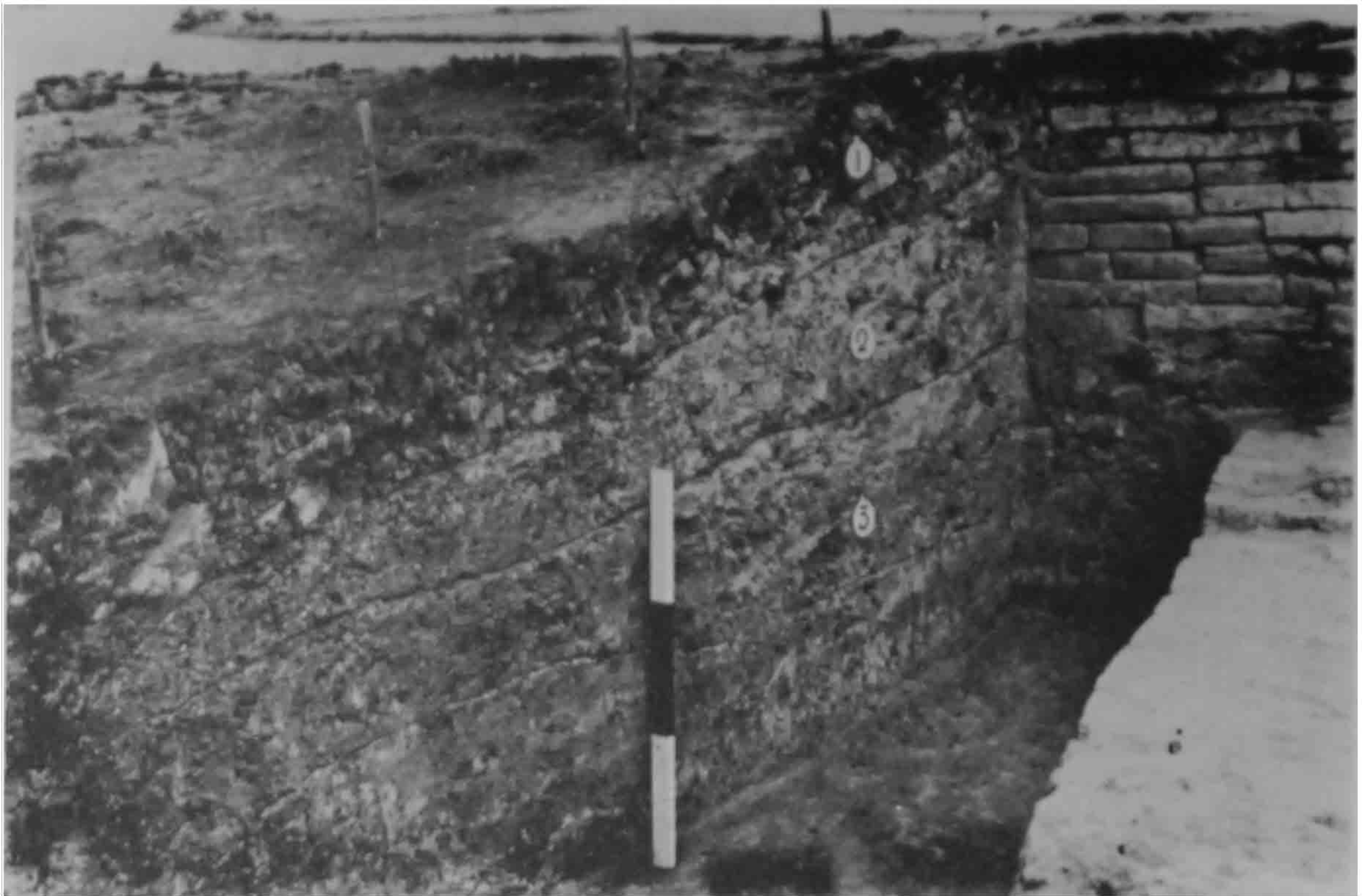
a. Part of Palace enclosure wall, KKG 25.
