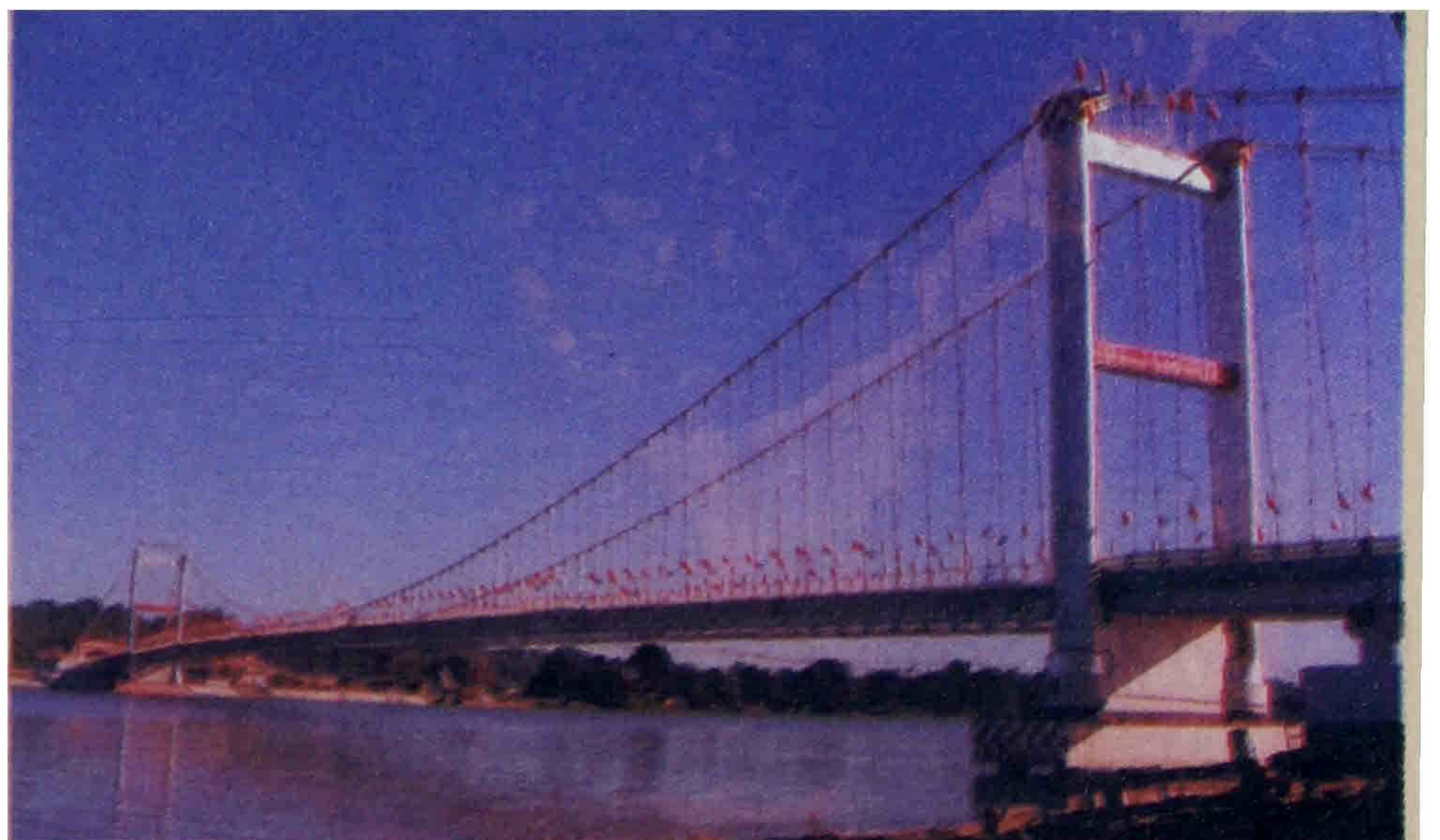
Ramoung Bridge, Rakhine
