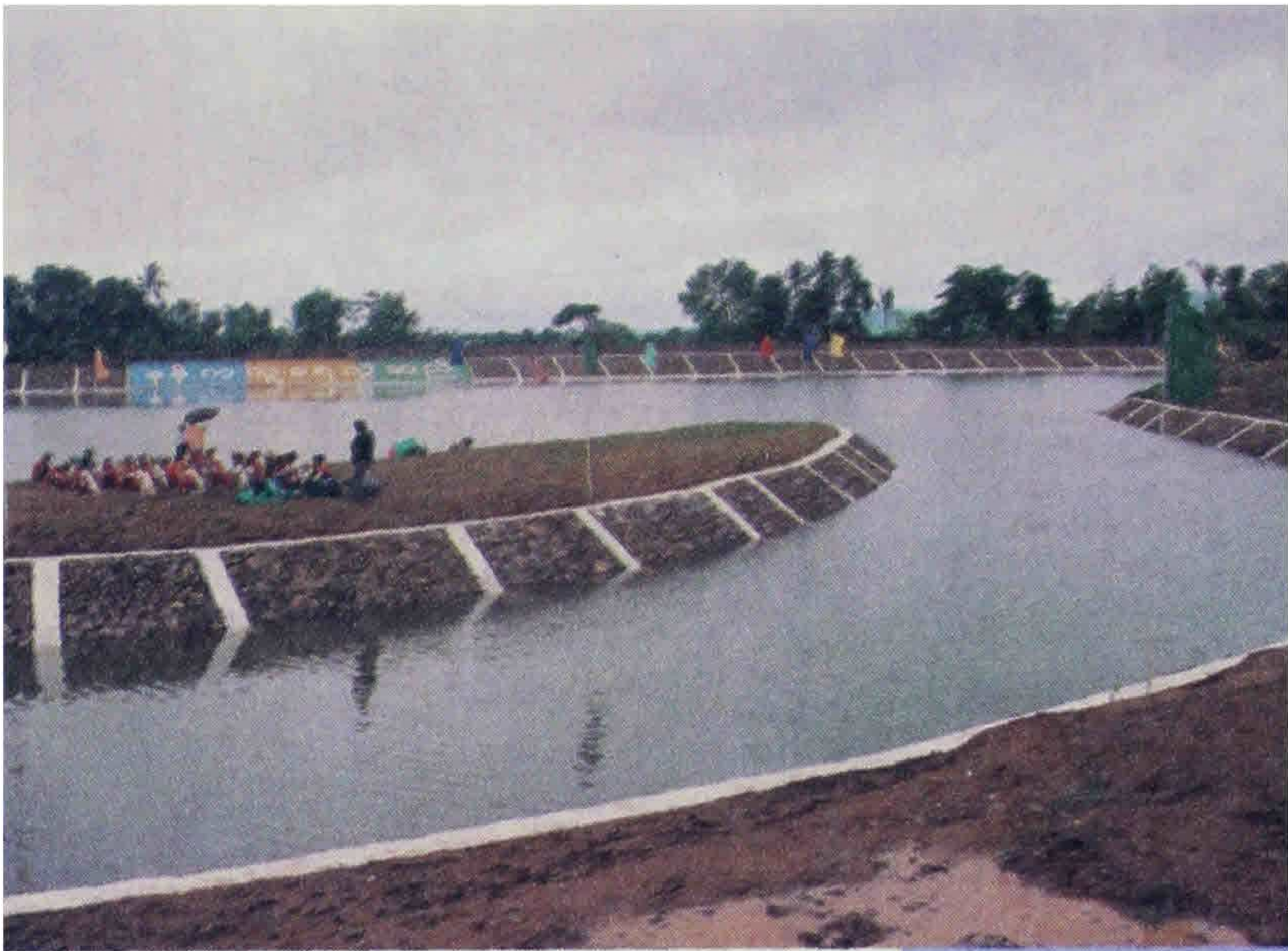
Nankathu Diversion Weir
