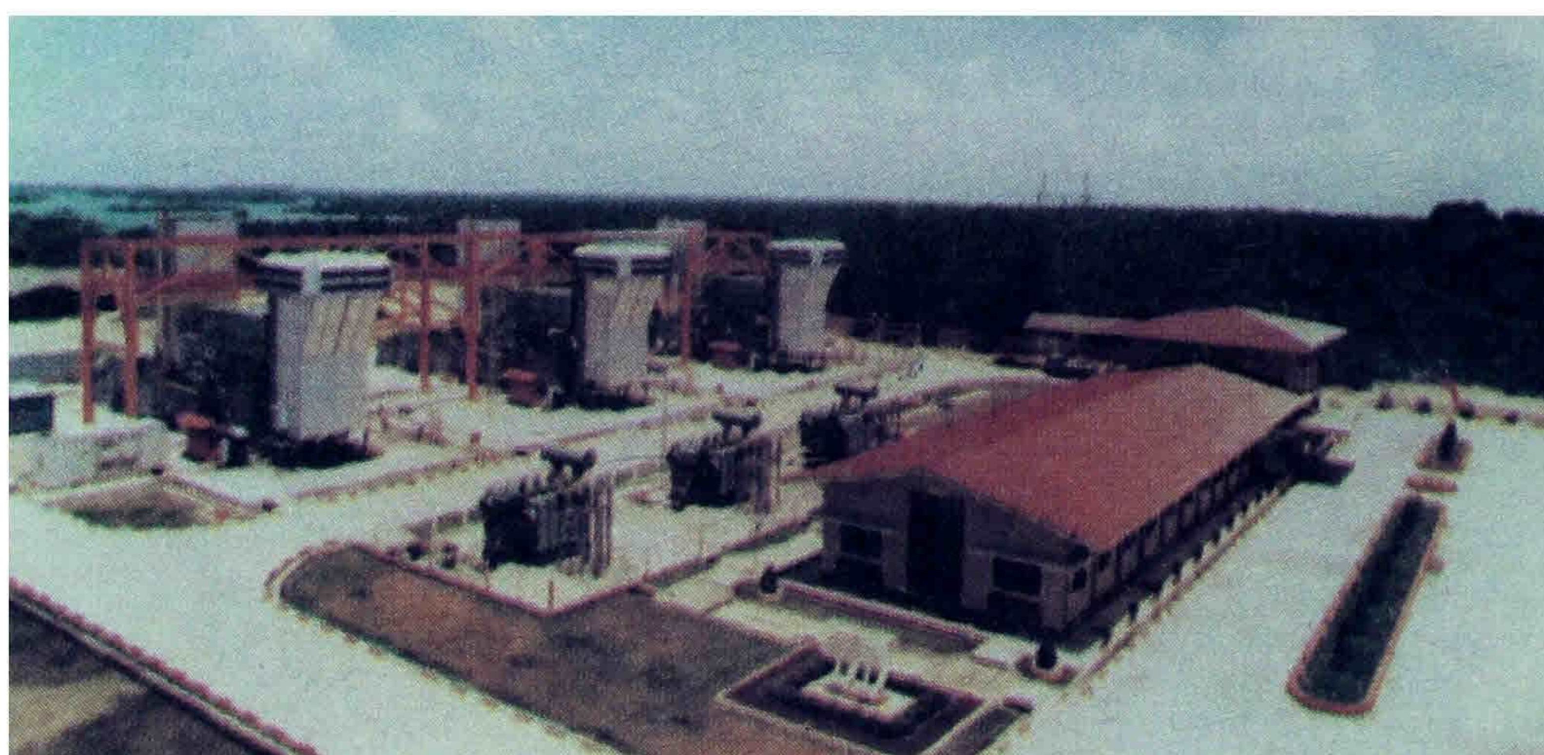
Hlawga Natural Gas Power Plant
