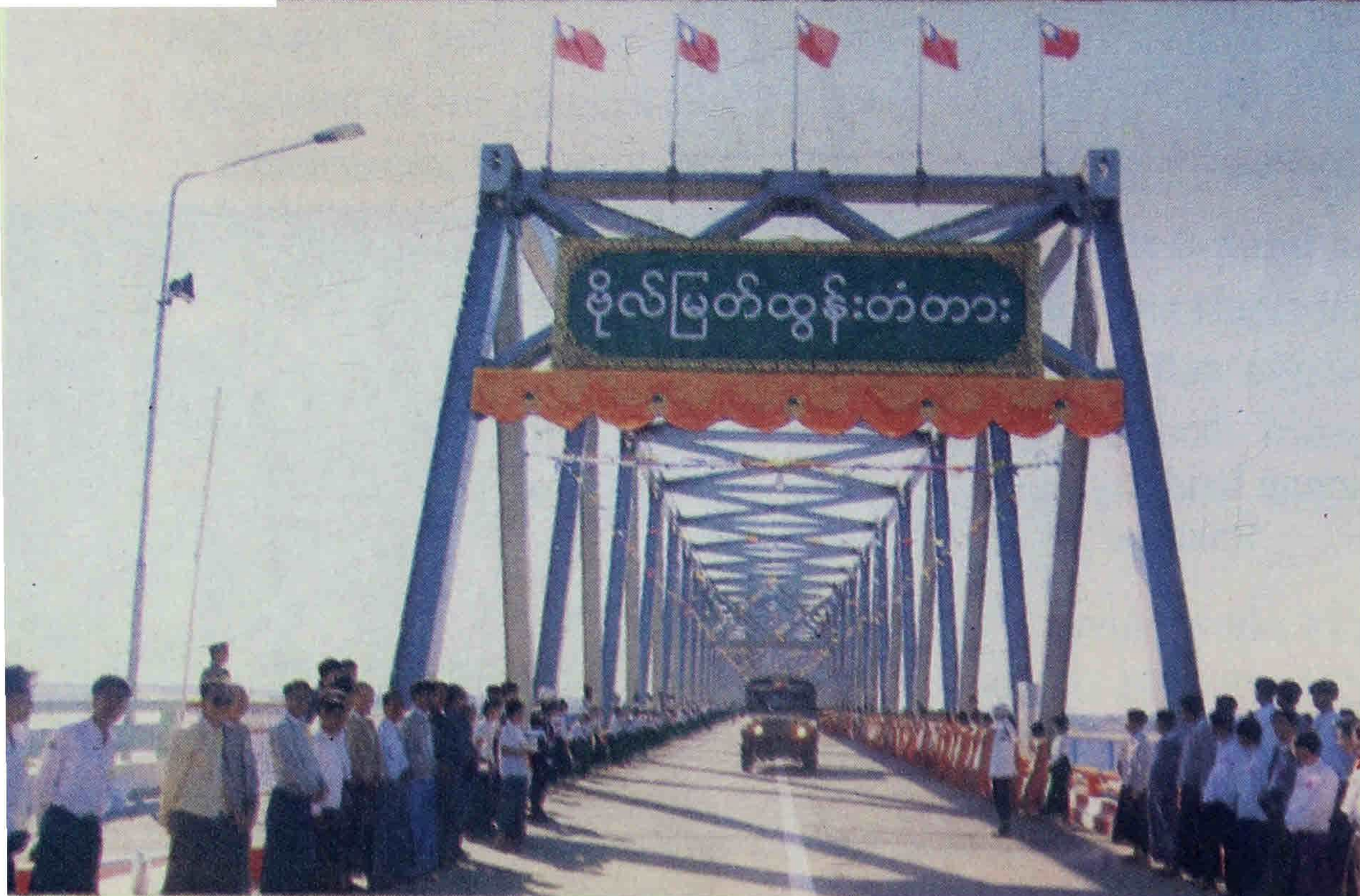
Bo Myat Tun Bridge
