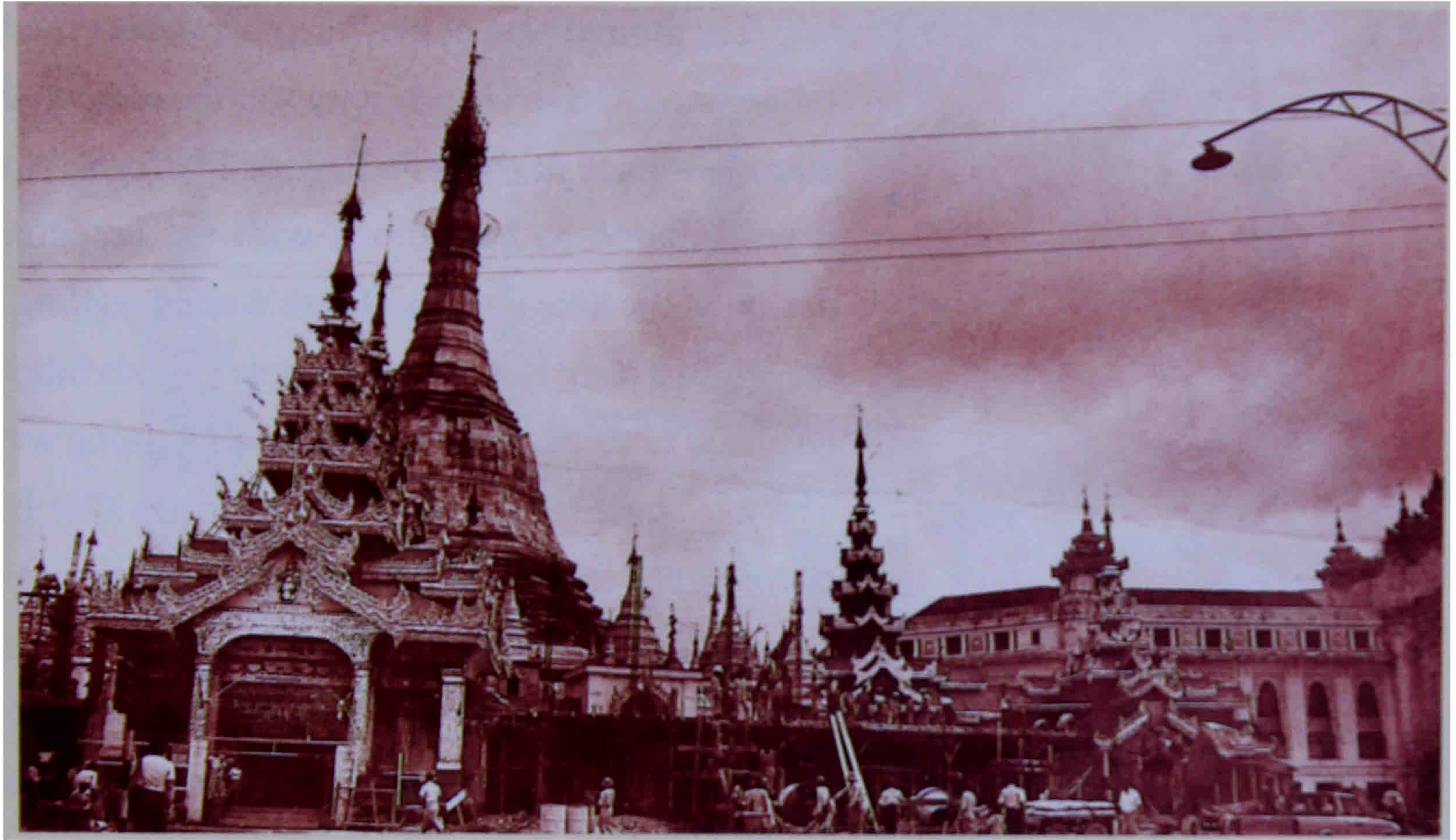
Non-stop renovation work at the Sule Pagoda under the overcast sky
