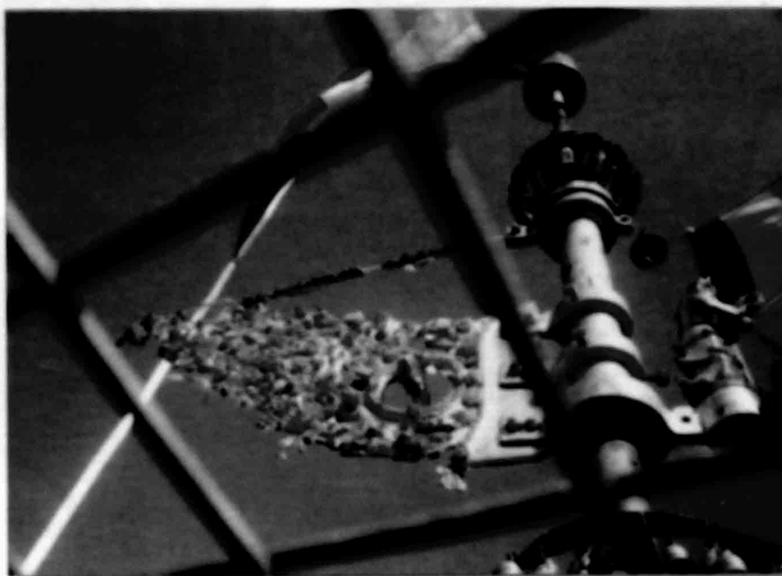
The vane and the figure of Sakka deity of solid gold used as a counter-poising weight ( plumb-bob ) against the vane
