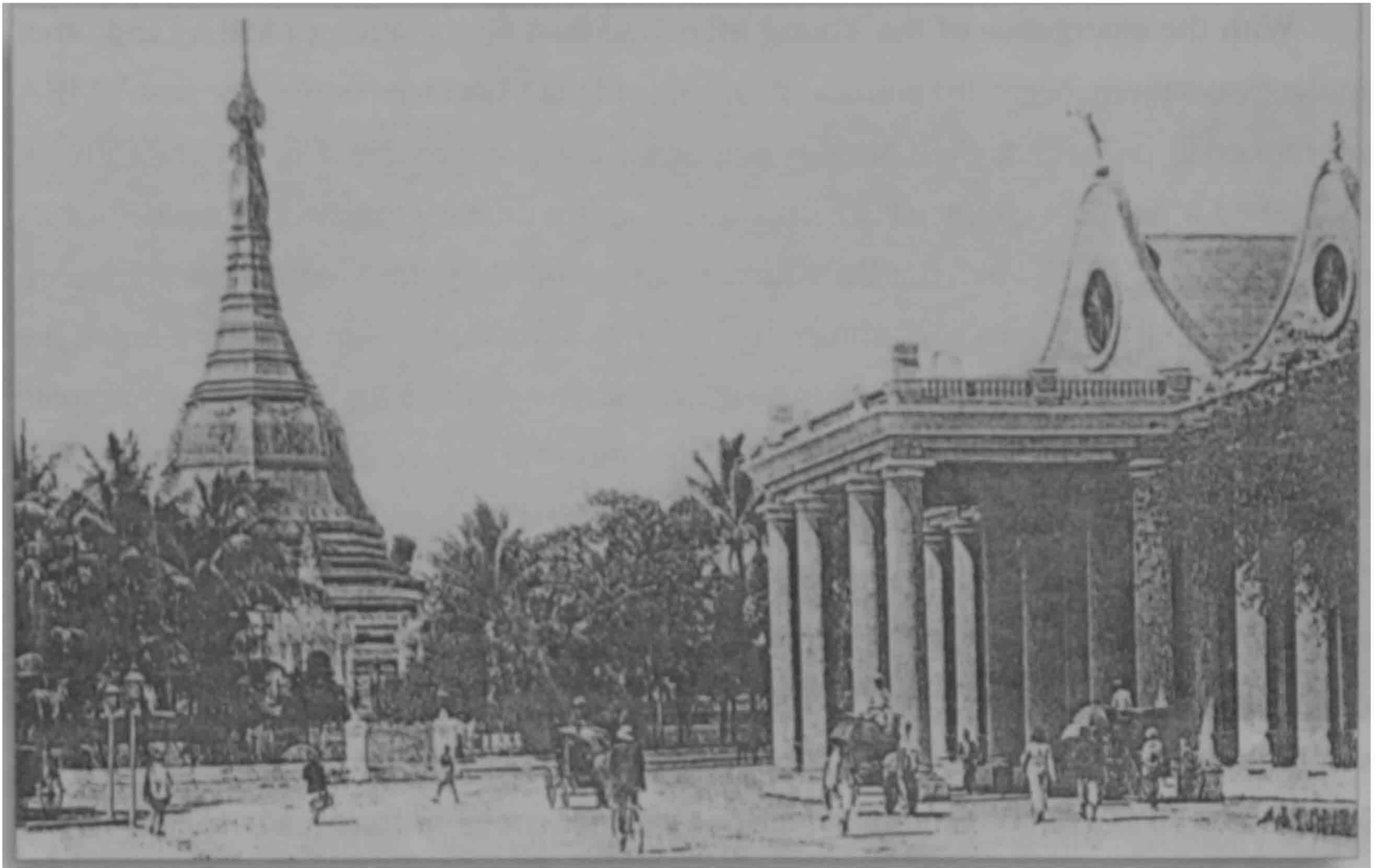
View of Sule Pagoda and former Town Hall
