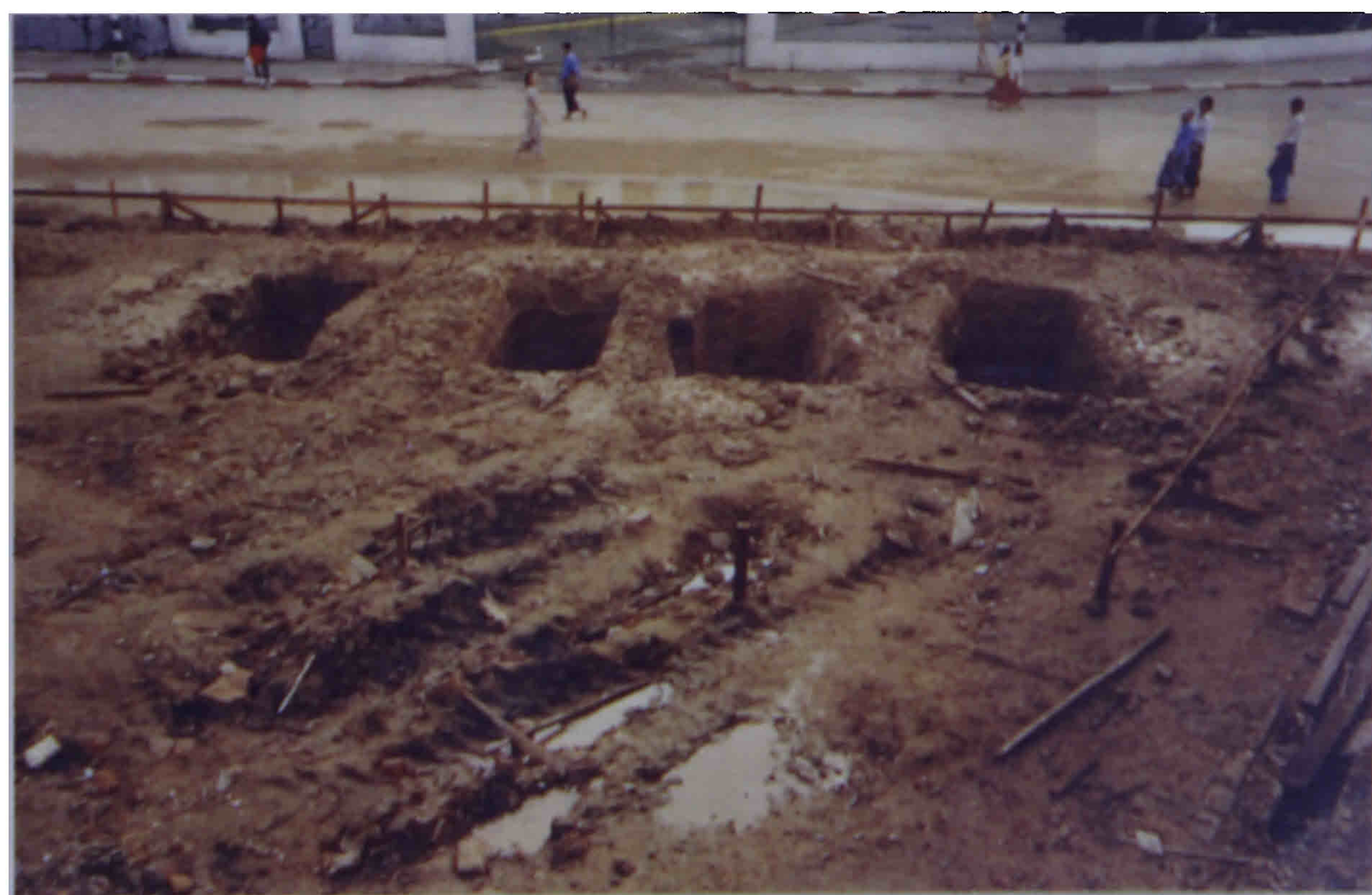
Preparation for ground-breaking ceremony at the Sunday Planet direction
