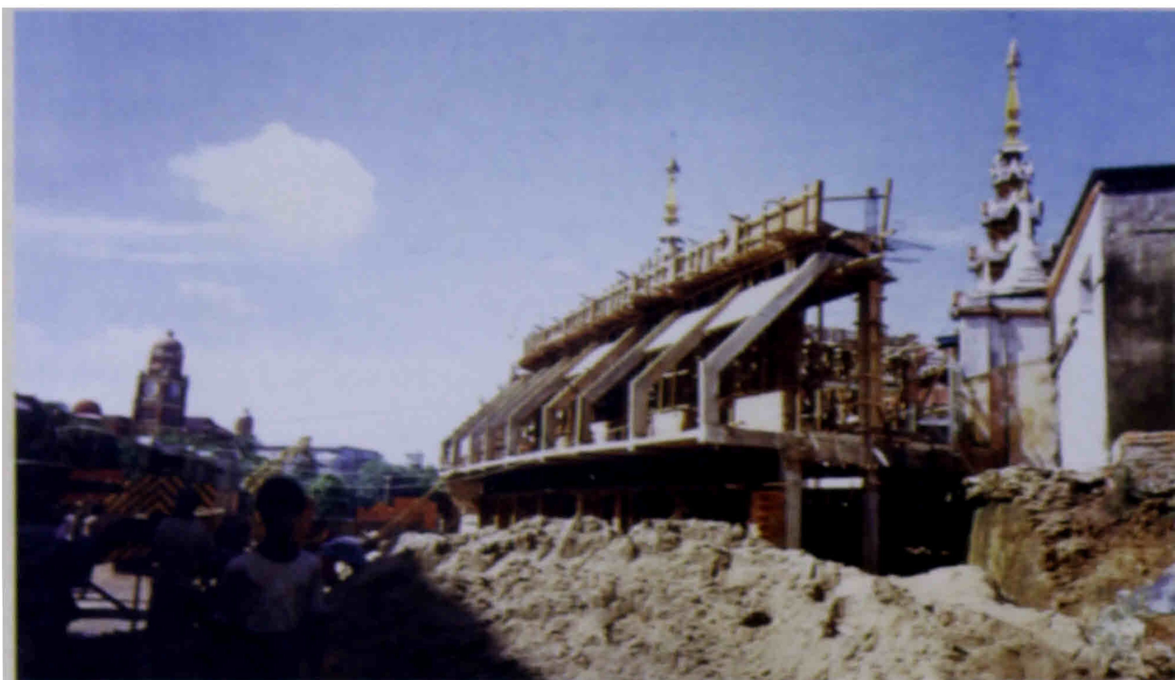
Progress in renovation work
