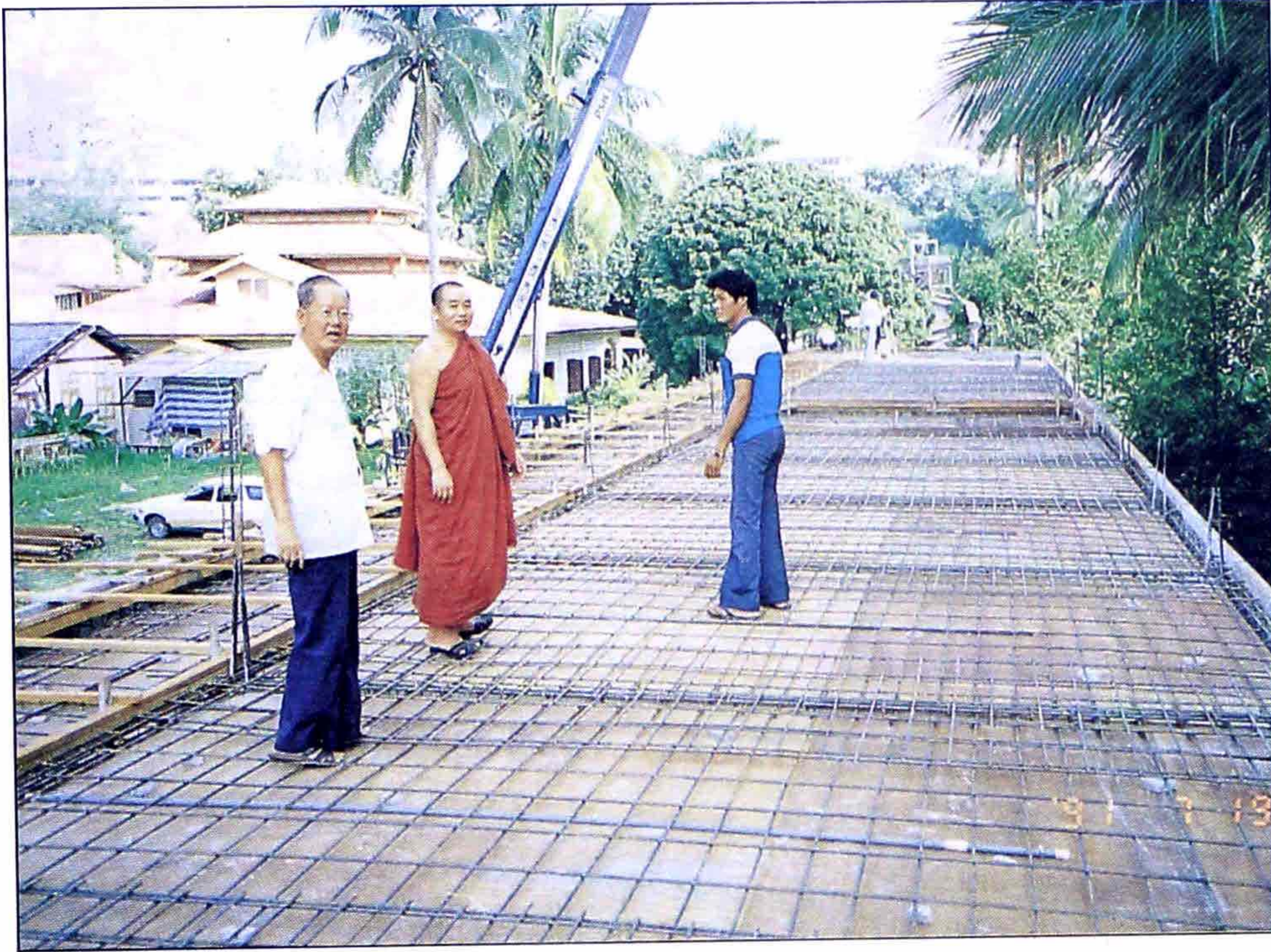
The Sila Bhavana Lodge building under construction
