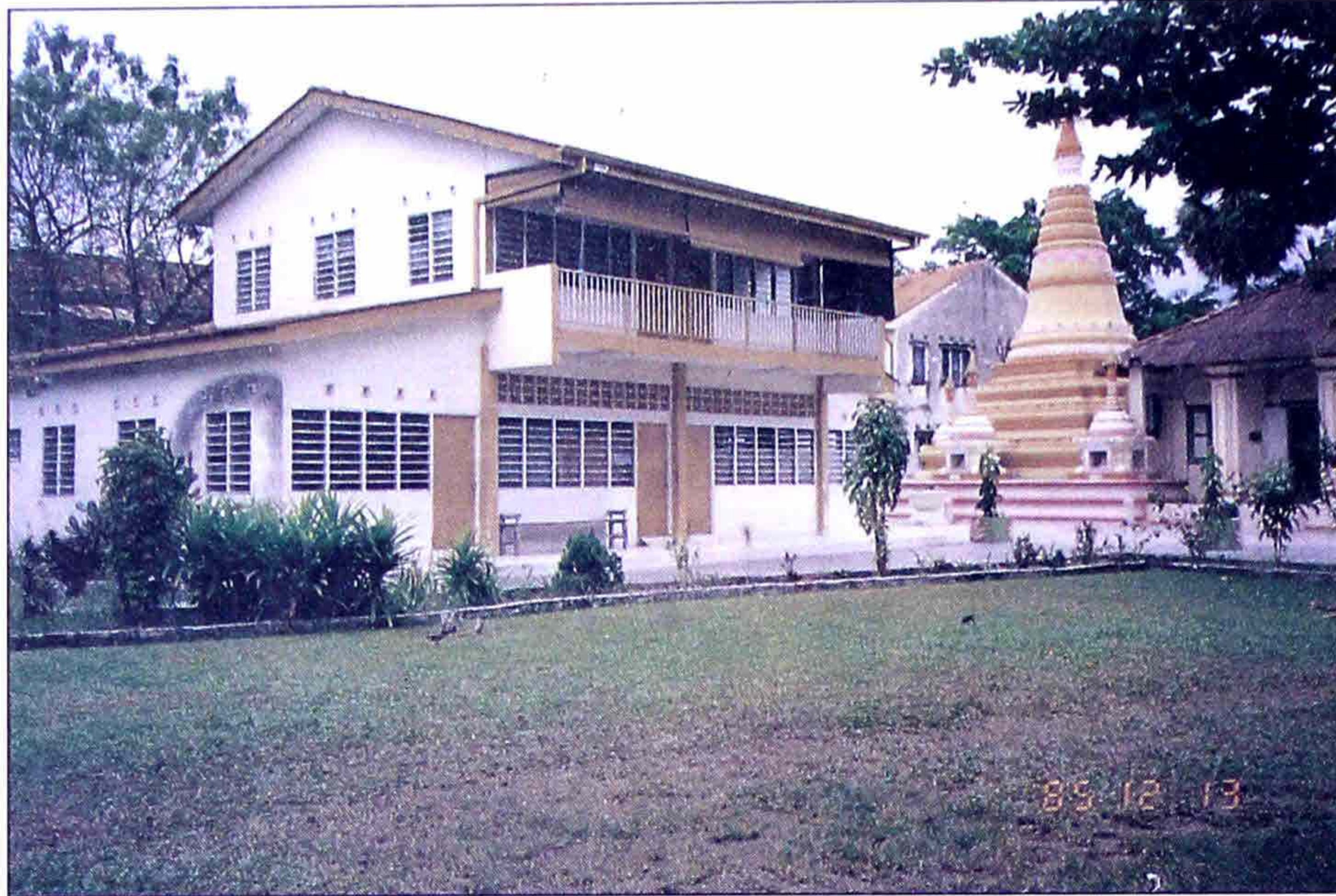
Sunday Dhamma School building
