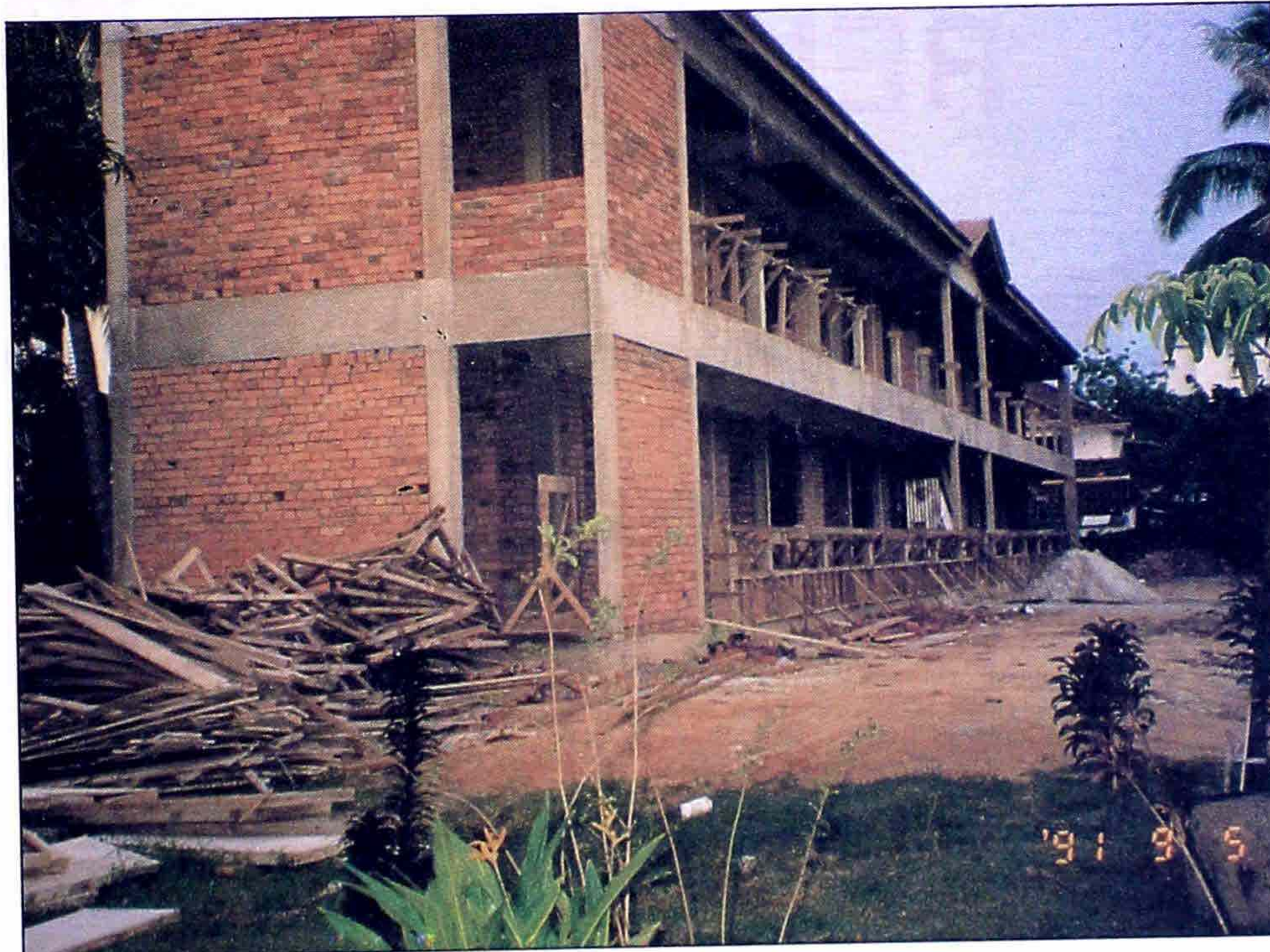
Almost completed Sila Bhavana Lodge building
